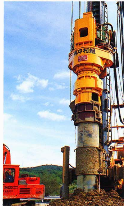
SMD-200H Pier expansion work steel pipe pile
