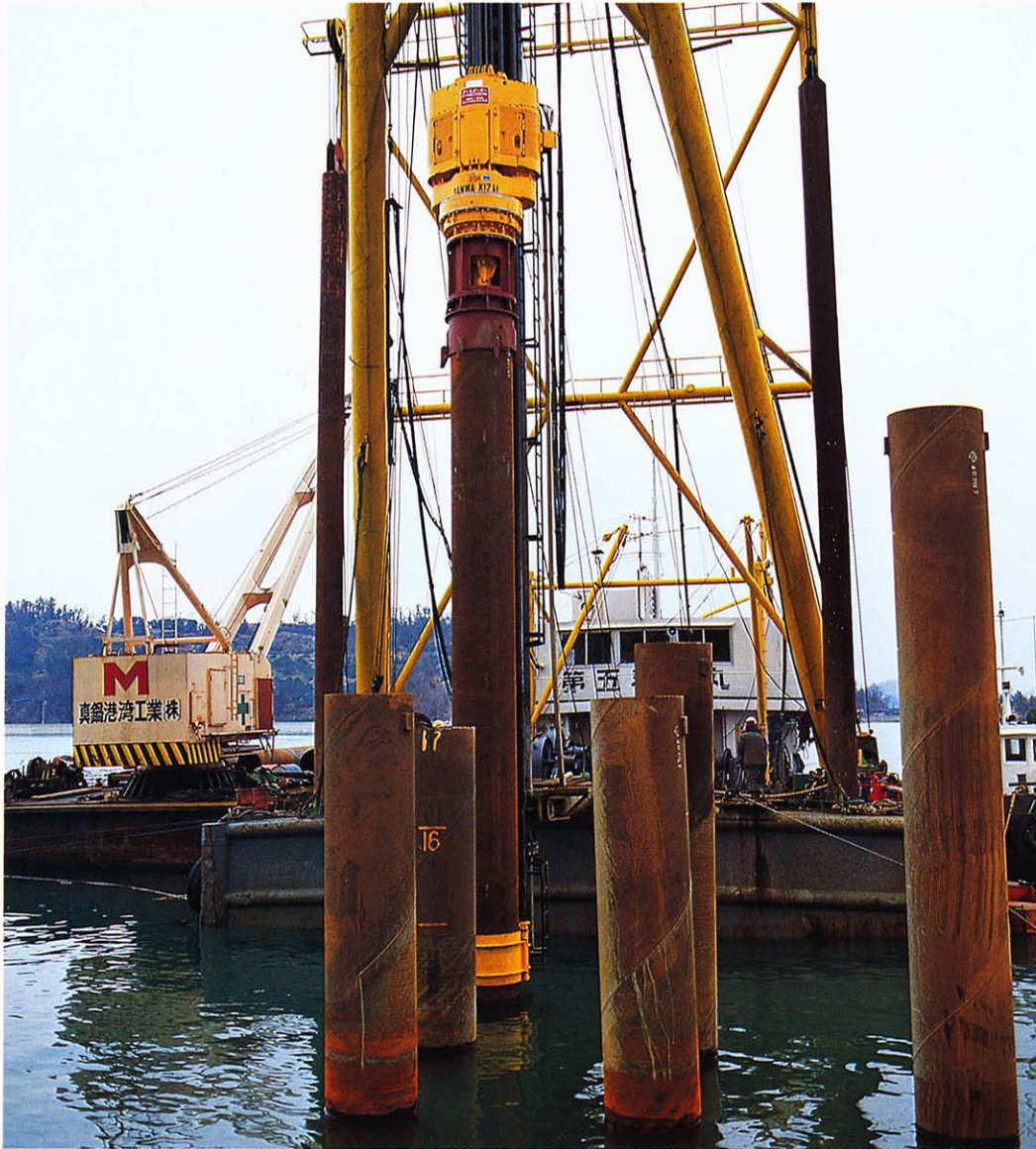
SMD-120H Embankment work steel pipe pile (800φ × 17M)
